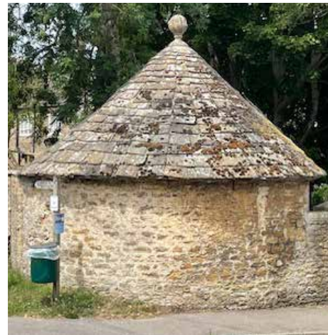
Fig 14a: The round building, possibly for drying wool, survives on the corner of Stubbs Lane
