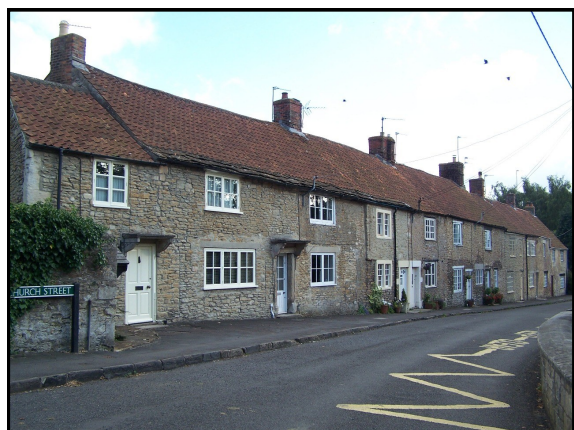
Unlisted Church Street row
