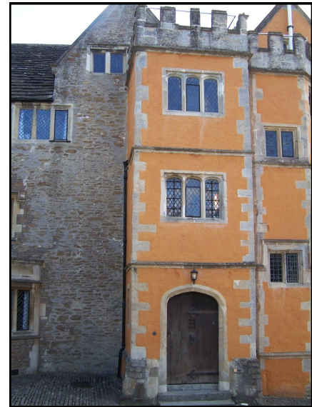
Porch and window bay of Beckington Castle
