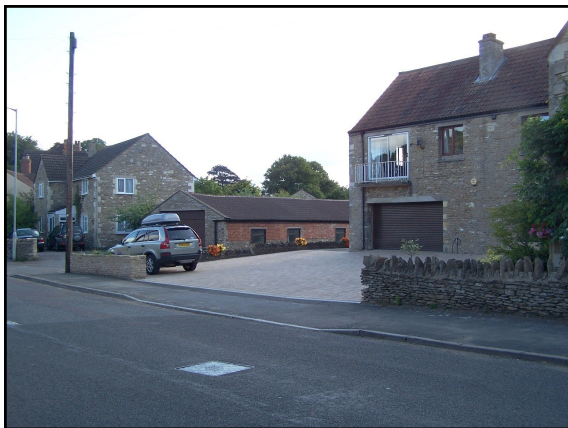
Loss of boundary on Bath Road
