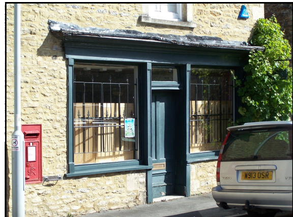
Shopfront, Warminster Road
