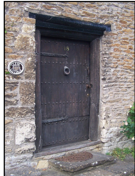
Planked door with rivet heads and strapped hinges at no.18 Church Hill
