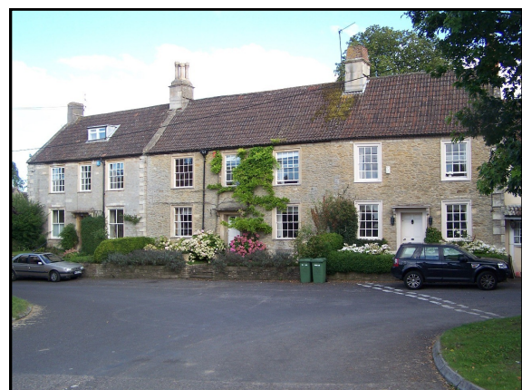
Typical sash windows at nos.19-23 Castle Corner
