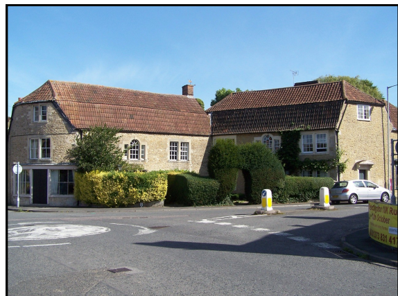
Pantiled mansard roofs on nos.1 & 3 Warminster Road
