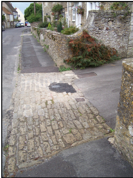
Stone setts on Goose Street
