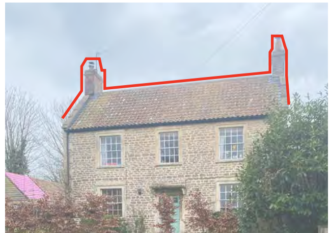
Figure 49: Traditional pitched roof with chimneys on gable ends on single detached dwellings
