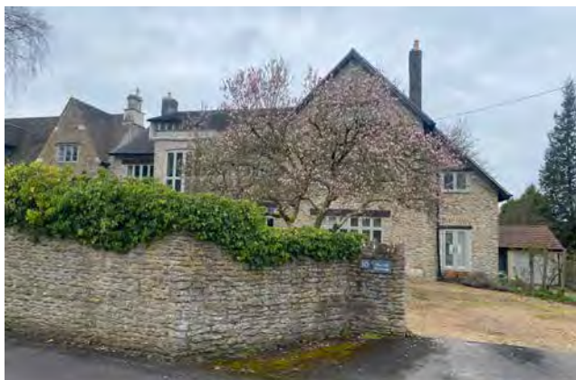
Figure 45: Stone wall combined with a hedge within the Conservation Area.
