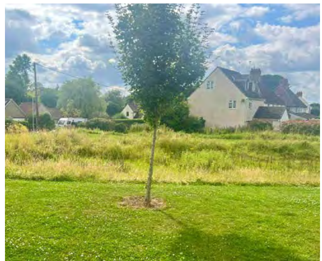
Figure 32: Example of Sustainable Drainage Systems that has been implemented in the Shepherds Way development.
