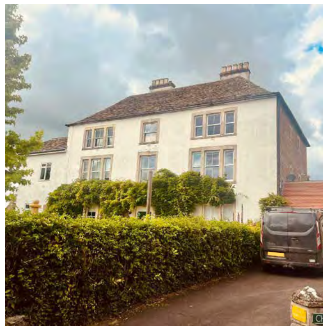
Figure 04: Springmead School, on Castle Corner.
