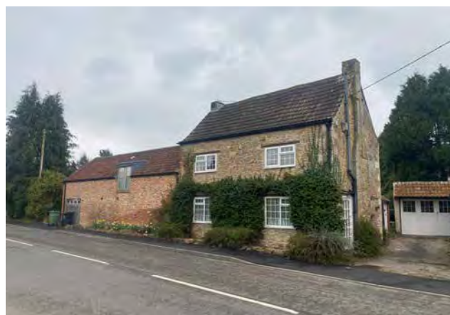
Figure 52: Detached building using traditional materials in Beckington.
