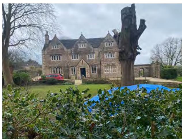
Figure 43: Beckington House, which is set back from Frome Road with a large front garden.
