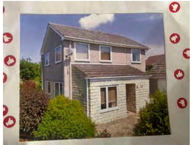
Figure 27: Example of building design (within the parish) that is not desirable.
